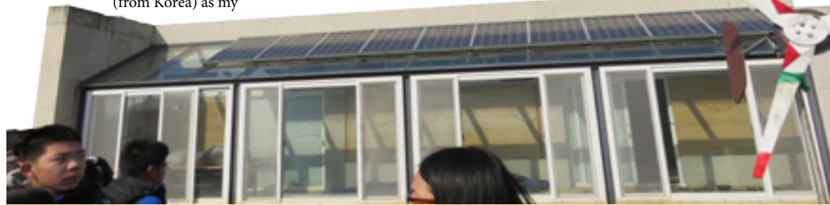
THE GREEN HOUSE. The passive house of the eco-village Galjeon of Sancheon uses energy from the sun. Photo by Geo Earl Angeles
